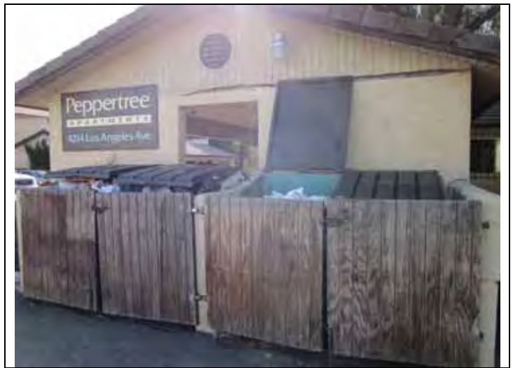
8. Waste disposal area at north side of the attached carport structure.
