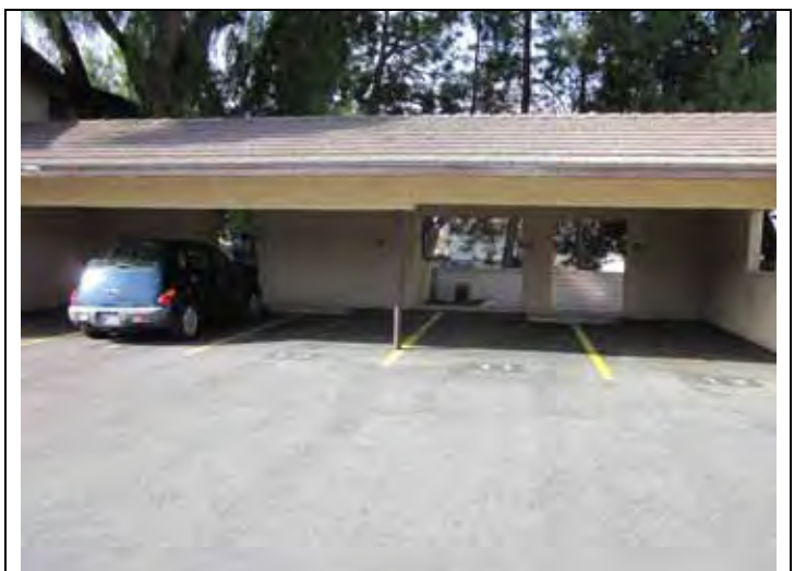
6. Attached carport structure.
