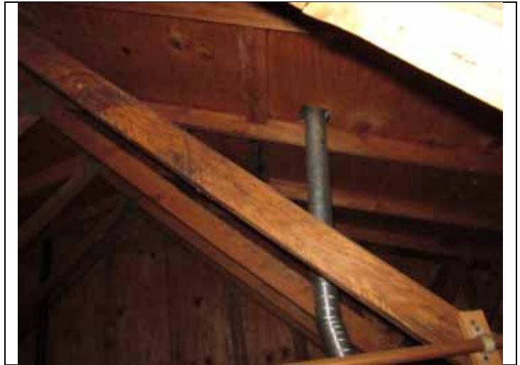
10. Attic and roof framing
